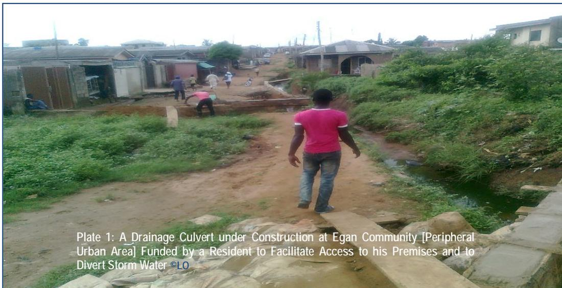
Plate 1: A Drainage Culvert under Construction at Egan Community [Peripheral Urban Area] Funded by a Resident to Facilitate Access to his Premises and to Divert Storm Water ©LO
